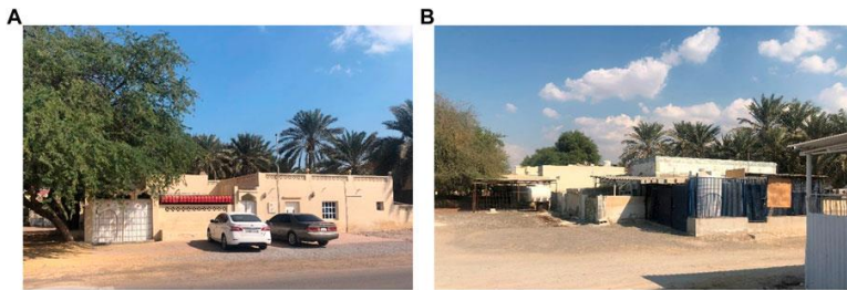
Figure 4: (A,B) Transformation of a Sha'abi house in Ras Al Khaimah shows its physical deterioration and many additions to the original layout of the house.
