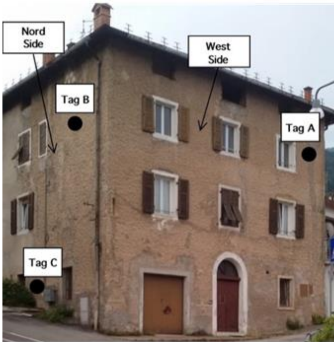
Figure 10: Photo of the considered experimental scenario, a 110 years old building under renovation.
